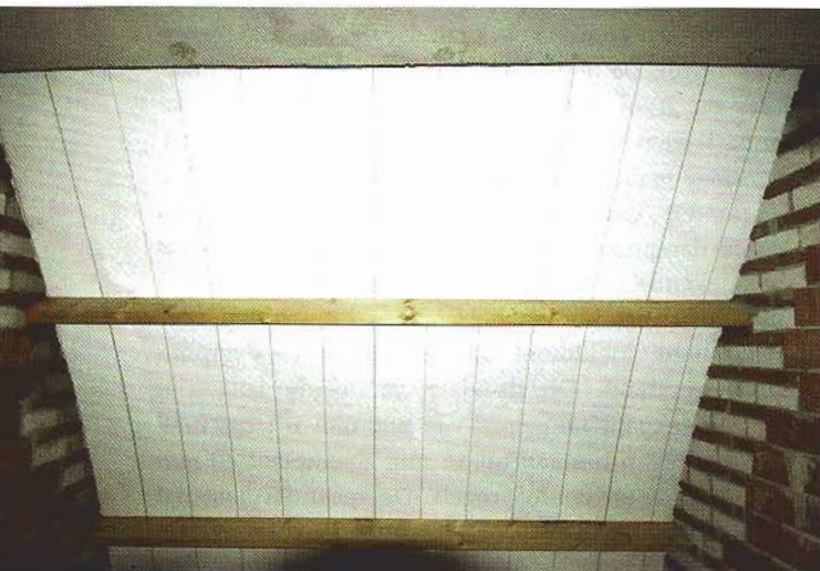
De binnenbeplating is schoonwerk.
